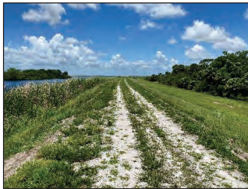
Photo 15 - North Reservoir. General View of North Levee.
