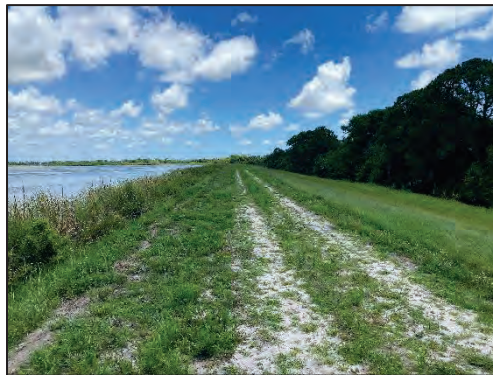
Photo 13 - North Reservoir. General View of East Levee.
