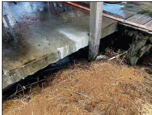
Photo 2 - South Reservoir - West Levee. Undermining Below the East Edge of the Pump Station Slab.
