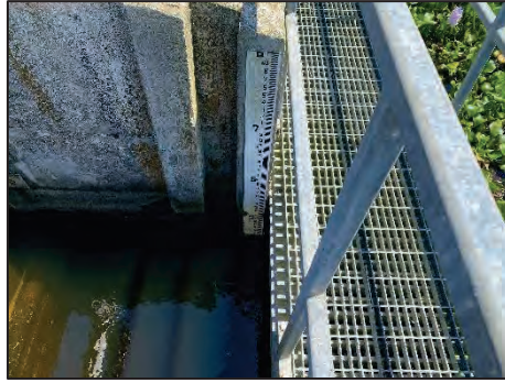
Photo 8 - South Reservoir. Water Elevation Gauge on Main Spillway.
