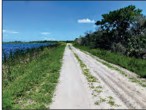
Photo 3 - South Reservoir. General View of South Levee.
