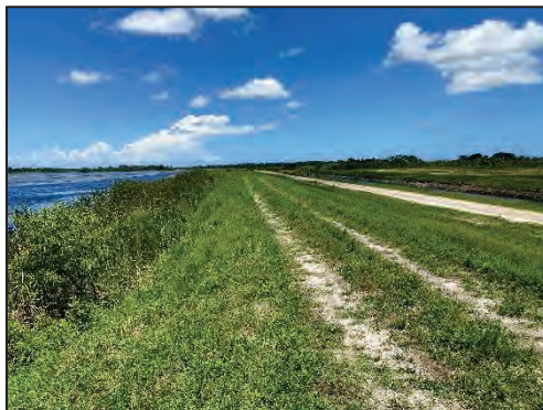
Photo 18 - North Reservoir. General View of South Levee.
