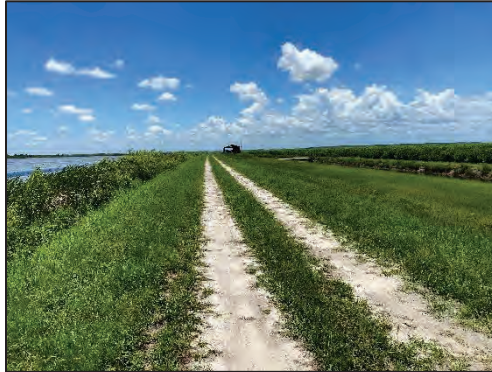
Photo 17 - North Reservoir. General View of West Levee.
