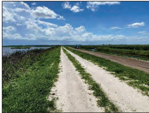
Photo 11 - South Reservoir. General View of North Levee.
