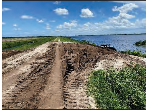
Photo 10 - South Reservoir. Levee Repair Area on North Portion of East Levee.
