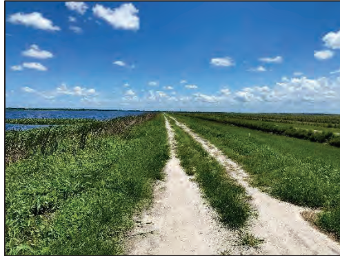
Photo 1 - South Reservoir. General View of West Levee.
