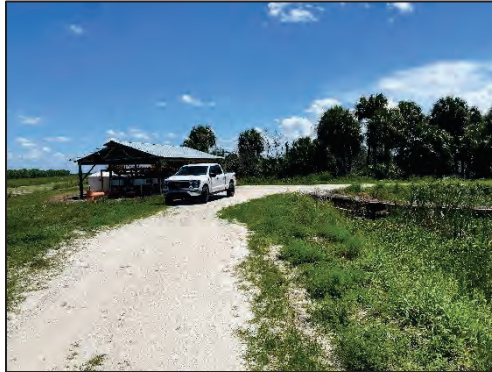
Photo 6 - South Reservoir – Pump Station at South End of East Levee.
