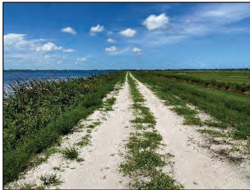
Photo 7 - South Reservoir. General View of East Levee.
