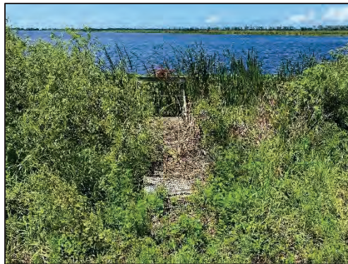
Photo 4 - South Reservoir. Wetland Supply Structure.
