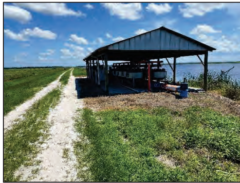
Photo 9 - South Reservoir. Pump Station Slab on East Levee.
