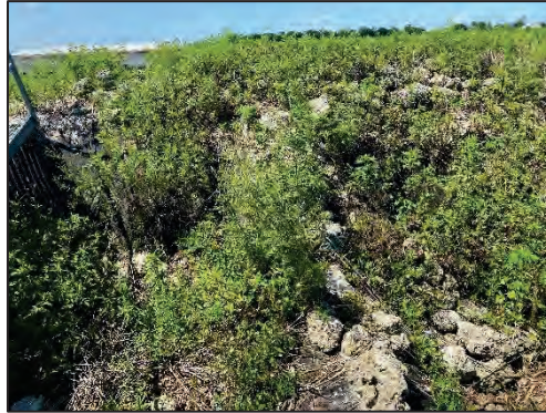
Photo 12 - South Reservoir. PS-1 Pump Discharge Pipe Location on North Levee.
