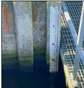
Photo 4 - South Reservoir. Water elevation gauge on main spillway.
