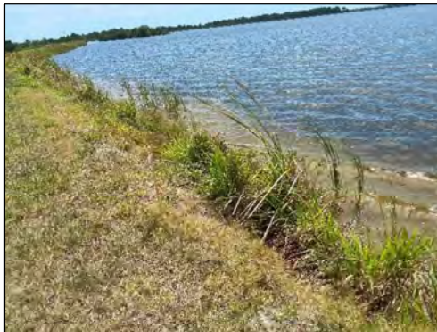
Photo 15 - North Reservoir. Bare Vegetation and Early Erosion Area Near Center of North Levee
