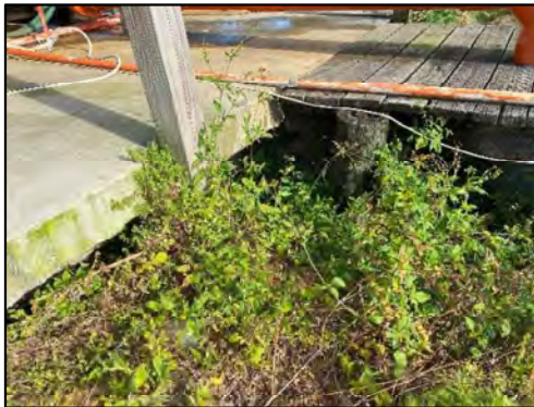
Photo 2 - South Reservoir - West Levee. Undermining Below the Pump Station Slab at Wooden Ramp
