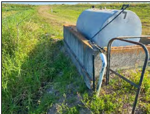
Photo 11 - South Reservoir. Undermining Below the Diesel Fuel Tank Slab
