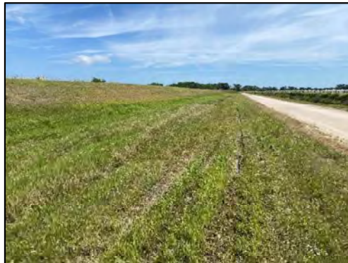
Photo 18 - North Reservoir. View of minor rutting near toe ditch on South Levee at the South Compartment.
