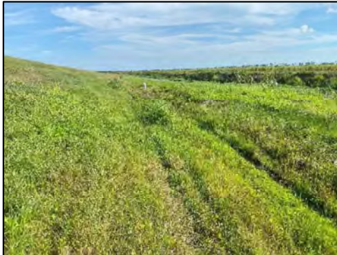
Photo 12 – South Reservoir – Rutting Noted Next to East Levee Toe Road
