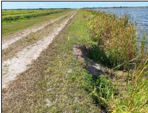
Photo 6 - South Reservoir. Erosion Area Just North of Area in Photo 5 (East Levee)
