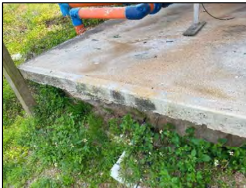
Photo 7 - South Reservoir. Undermining of Pump Station Slab on East Levee
